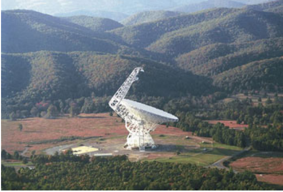
The Robert C. Byrd Green Bank Radio Telescope (GBT) focuses 2.3 acres of radio light. It is 150m tall, nearly as tall as the nearby mountains and much taller than pine trees in the national forest. The telescope is in a valley of the Allegheny Mountains to shield the observations from radio interference. (Image: NRAO/AUI)
