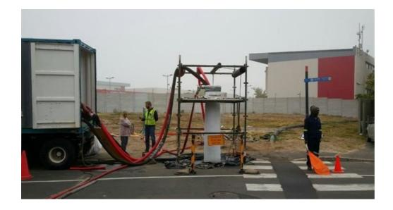
"A safe installation was implemented through excellent coordination and communication, with minimal impact and disruption to the public. The end result was a set of seven cost-effective, well-cured and rehabilitated close-fit lined sewer sections, with a total length of over 700m. The project was also achieved well within the programme schedule of the overall contract," Röhrs highlights.
