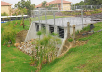
The rainwater is collected and stored in an underground dam on the Vodacom premises. (Image: Vodacom)
