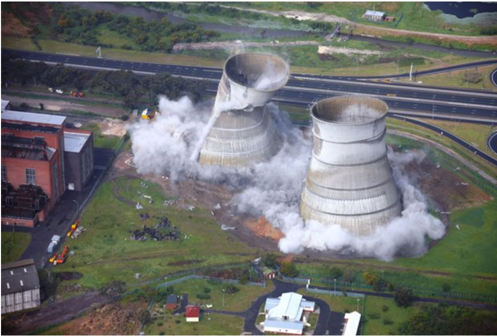
Controlled implosion of redundant cooling towers. Image supplied
